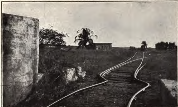
A. Subsidence of the ground with consequent tilting of buildings in the Victoria Battery, Port Royal. The kink in the railway track is over a fault.
